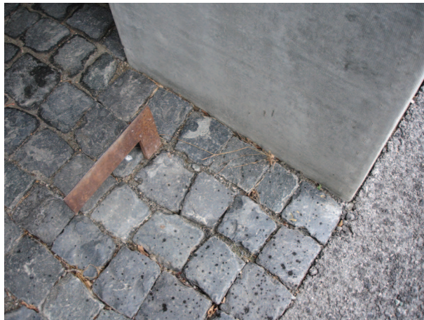
Figure 6. Consistent, beautifully-cast concrete. Photo: Christopher Platt.
