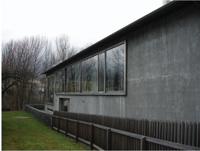
Figure 9. Window frames hang picture frame-like, similar to those in the Kolumba museum (below). Photo: Christopher Platt.
