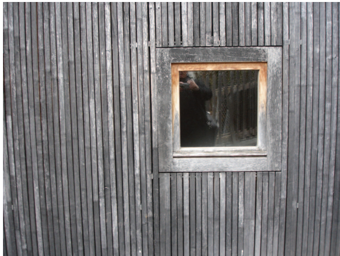
Figure 4. Narrow, weathered larch cladding. Photo: Christopher Platt.
